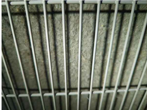
Close up of compressor fins clogged with dust and debris
