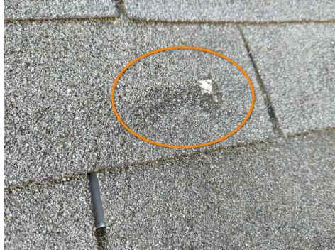
Damaged shingle
