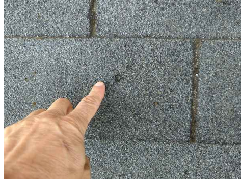
Damaged shingle
