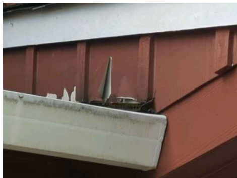
Front, over walkway
